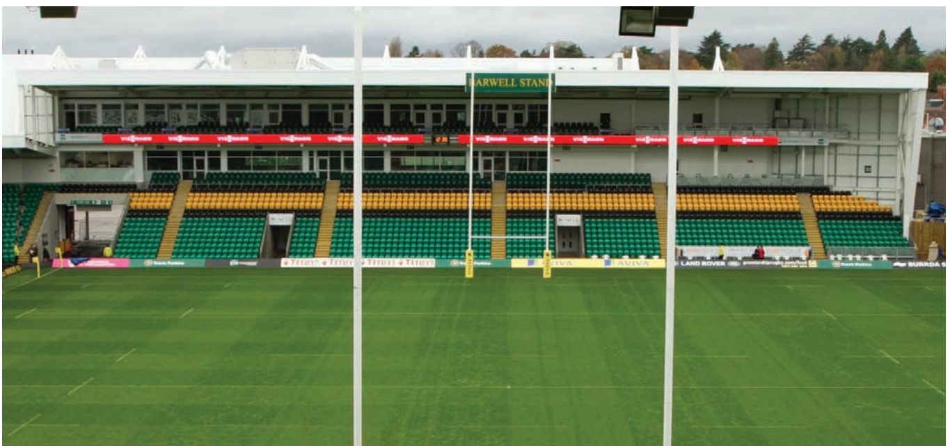
Construction of the Barwell Stand took seven months
